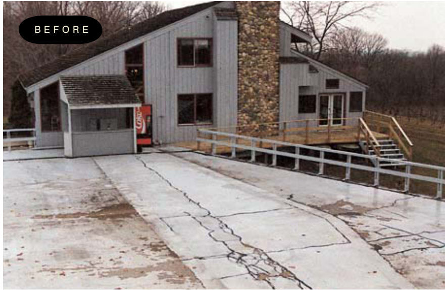
LEAKING, UNSIGHTLY ROOF OVER WINERY
